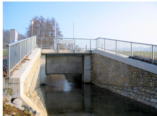
Design: TESACO, acc. to DIN 19569-4, BS 7775:2005, ANSI/AWWA C561-04, 4-face sealing
